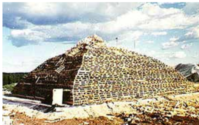
Figure 6.1: Leachate evaporation pyramid at Hogbytorp landfill, Sweden
