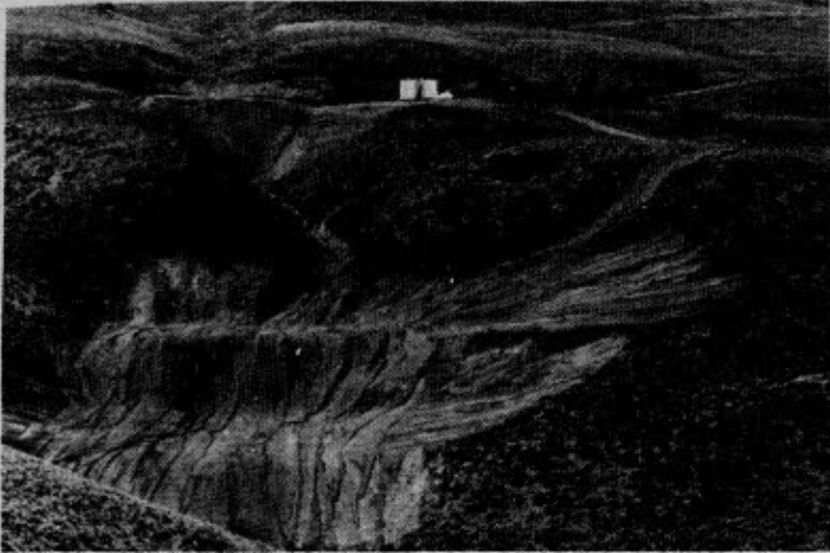
1. & 2. This is a drilling location and gas well. The bulldozed area in the foreground was once the mud pits, constructed in the bottom of a water-course. Into the mud pits went the drilling mud, caustic soda, fracturing oil, and other toxic chemicals used in well completion. When the pits overflowed into the spring-fed, wooded draw below, a 2" to 12" layer of waste material was deposited for approximately 1 1/2 miles downstream. It is shown in the photo below. The mud pits served no purpose, but 6-8 acres were denuded and exposed to erosion. No revegetation is required by Wyoming or Federal law. In addition, this gas well free-flowed to the atmosphere for almost a week, killing 2-3 acres of vegetation downwind. One gas well has resulted in surface destruction of approximately 13 acres at just one site alone.
