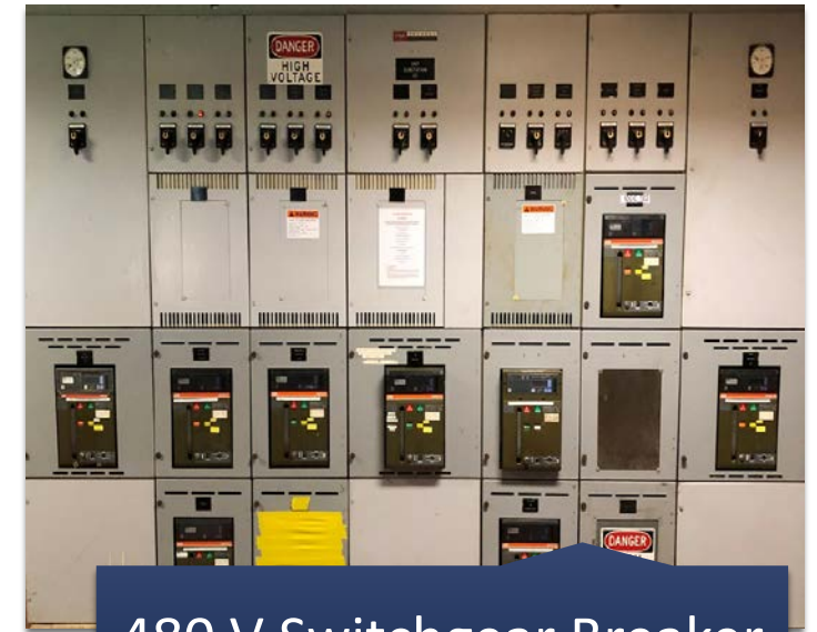
480 V Switchgear Breaker Replacement (Phase 2)
