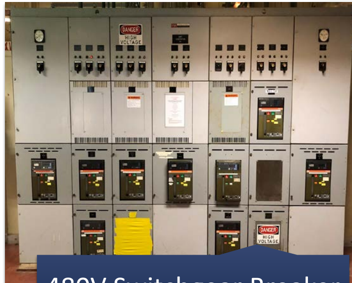
480V Switchgear Breaker Replacements (Phase 1)
