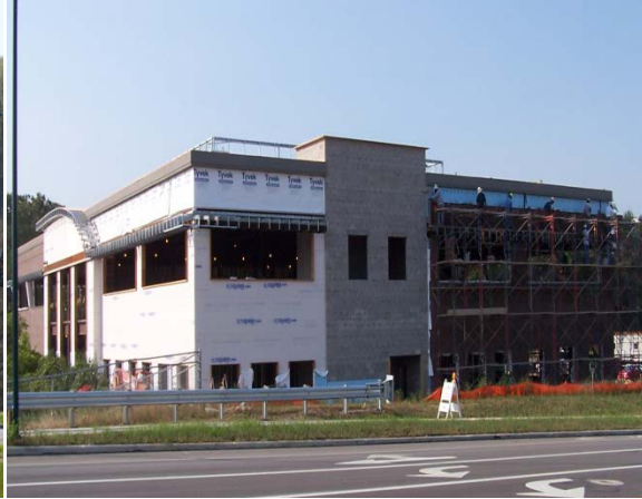
Central Ohio Urology Group Under Construction
