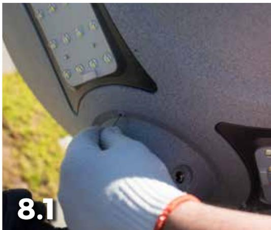
**TIP:** If you misplace the lamp pin key, you can also use a paperclip.
