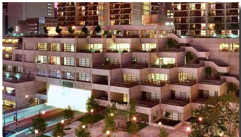
Agape Senior Center (Angelus Plaza in Los Angeles, CA) will begin a $3 million rehabilitation project in 2014.
