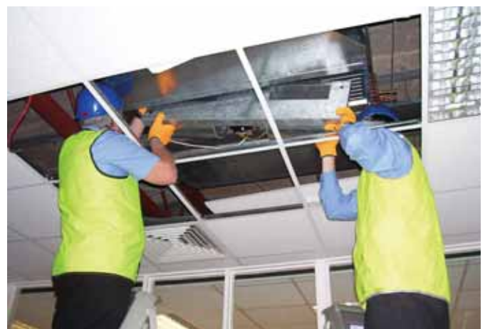
Figure 7.1 Replacing a fan deck in a large fan coil unit
