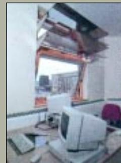
At APU, the twin internal light shelves of semi-transparent reflective glass have proved ineffective in enhancing light levels deep into the space, as the daylight is reflected into the coffers of the waffle slab ceiling.
