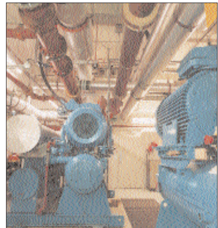
The ammonia chillers are only used as peak lopping devices for a few days a year.
