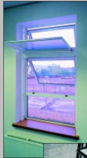
Occupants liked the upper motorised window, but the central window elements close under only a small wind, leading to...
