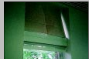
A makeshift anti-glare control for some of the west-facing windows.
