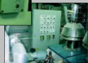
...but thumbs down for placing the summer/winter switch at the end of a plantroom obstacle course.
