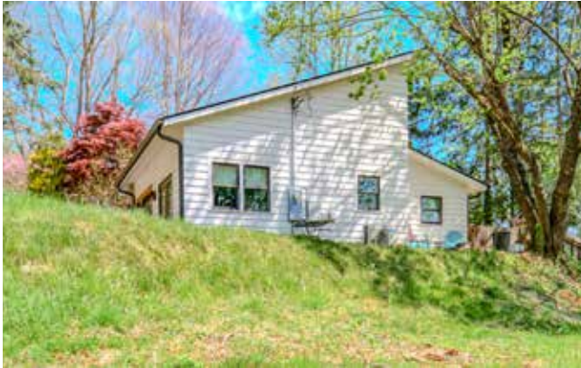
Side View of Suite, Leading into Yard
