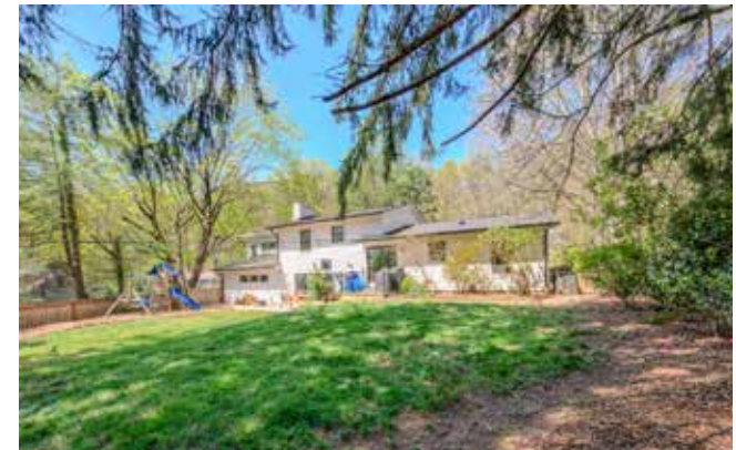
Rear View of Home from Yard
