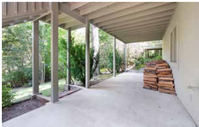
Dry Storage under Front Porch
