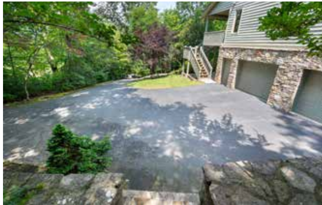
Exterior Paint Completed in 2024
