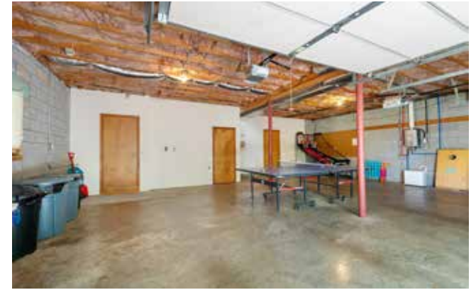
Garage Storage Area
