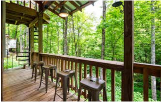
Spiral Stairs Lead to Bonus Space or Storage
