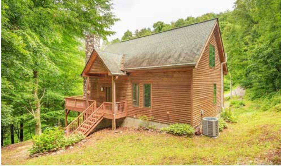
Spring photo — new roof was added December 2023
