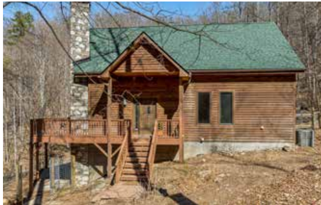
New roof added in 2023
