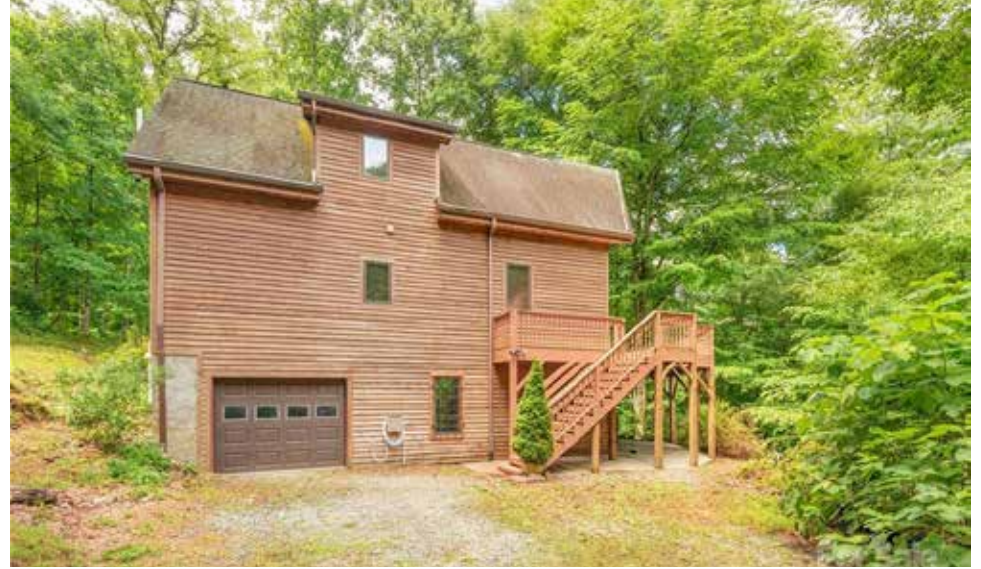
Spring photo — new roof was added December 2023
