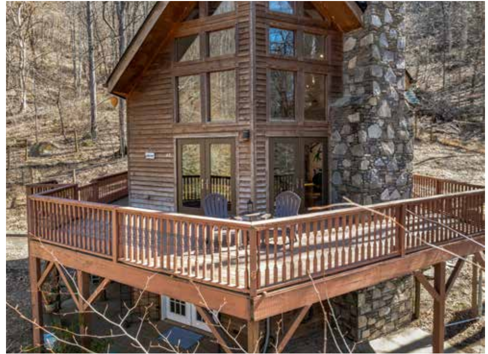
Floor-to-ceiling windows showcase the amazing views!
