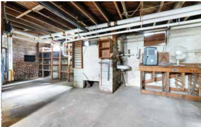
Large, Unfinished Basement
