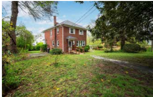
New Roof, Gutters, and Gutter Guards in 2023
