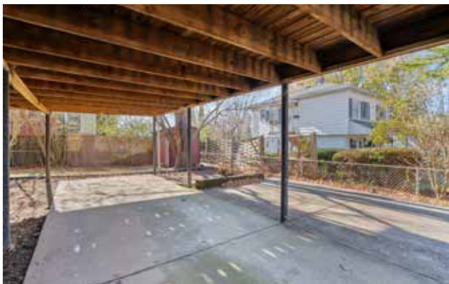
Another Angle of the Carport
