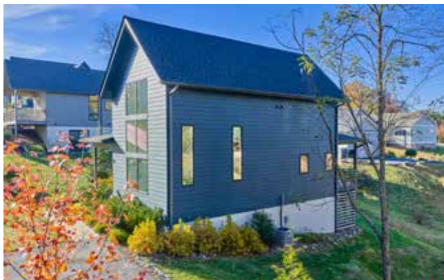
Enclosed Storage Below Deck
