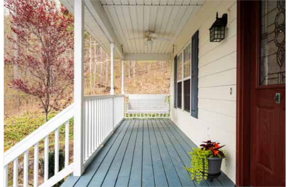
Covered Front Porch
