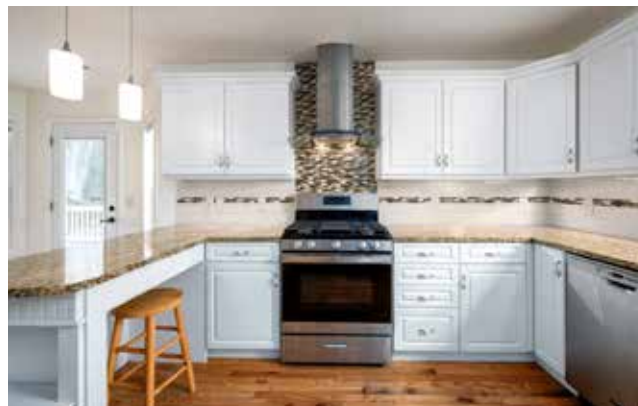
Gas Oven/Range with Exhaust Hood
