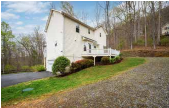
Side View of Home Showing Garage/Drive
