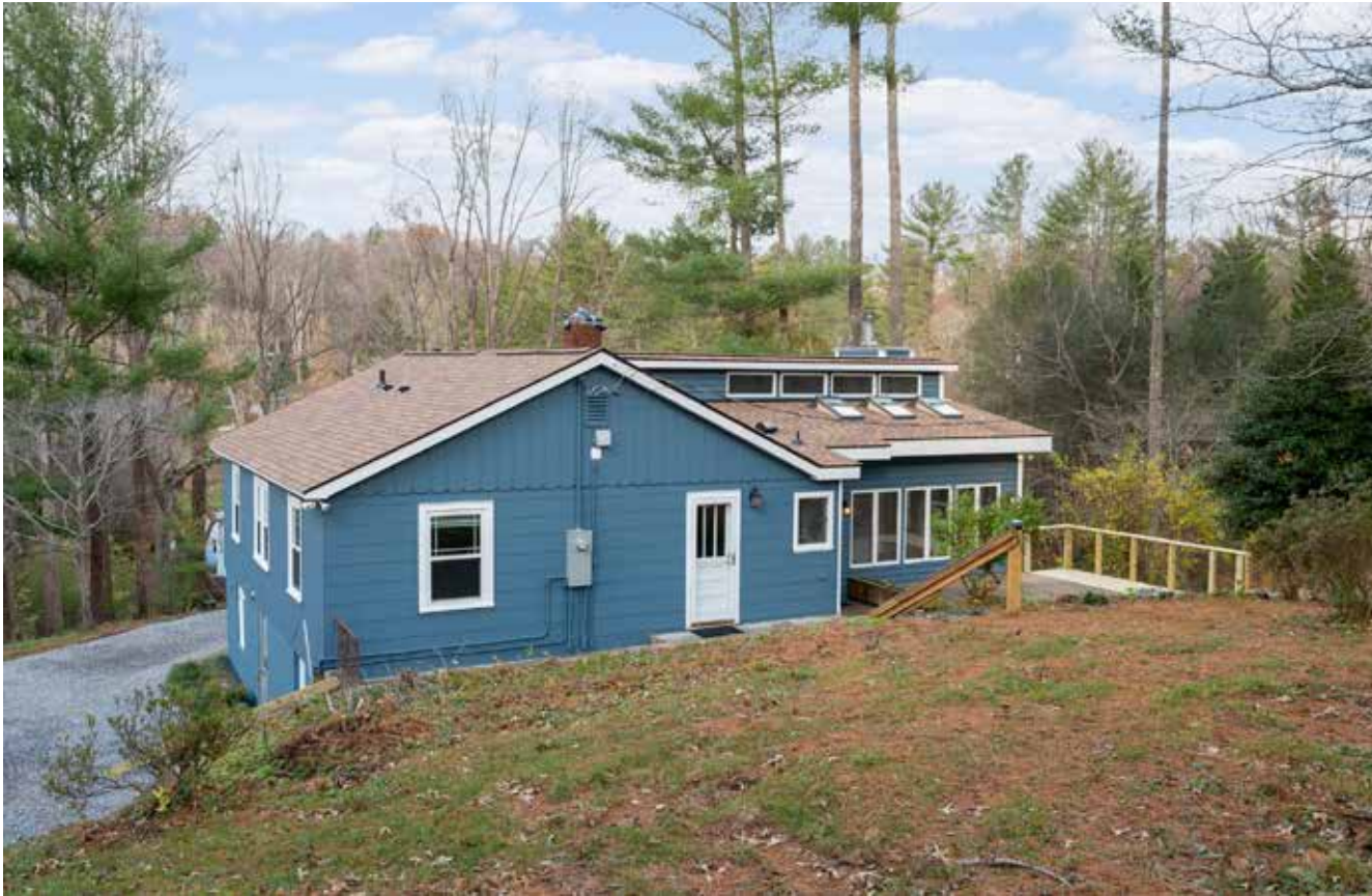
Home's Exterior Was Professionally Painted, Including Trim, Soffits, and Fascia
