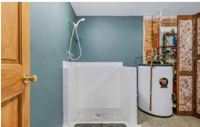
Doggie Shower in Utility Room
