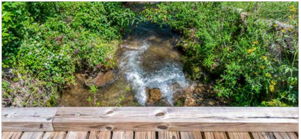
Roaring Fork Creek Bridge
