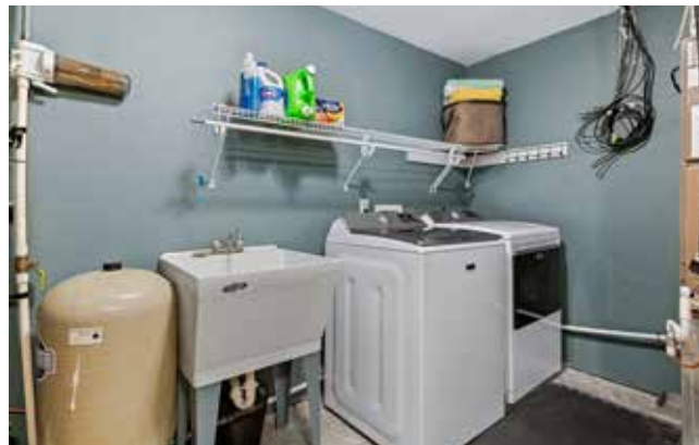
New Washer and Dryer Convey
