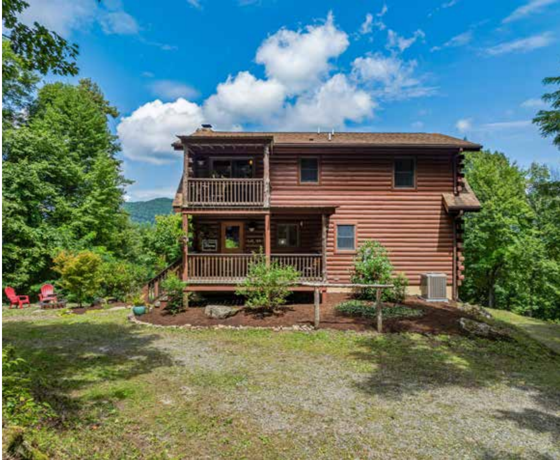
Entrance to Main Level and Parking Area
