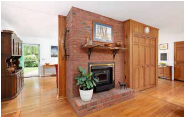
Wood-Burning Stove Has Been Regularly Serviced
