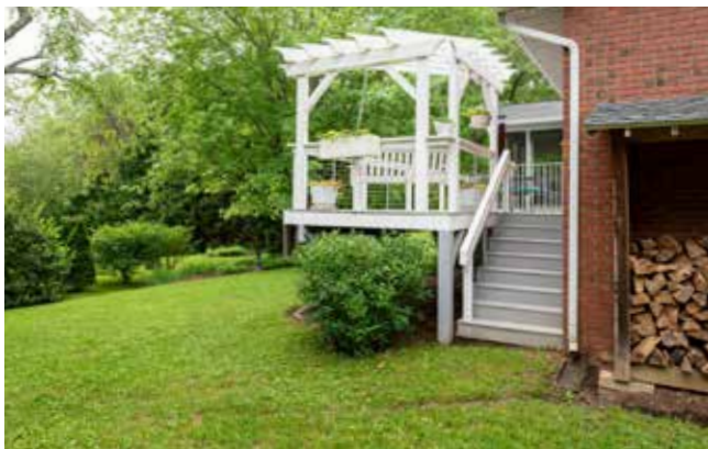
Firewood Storage Is Just off the Deck
