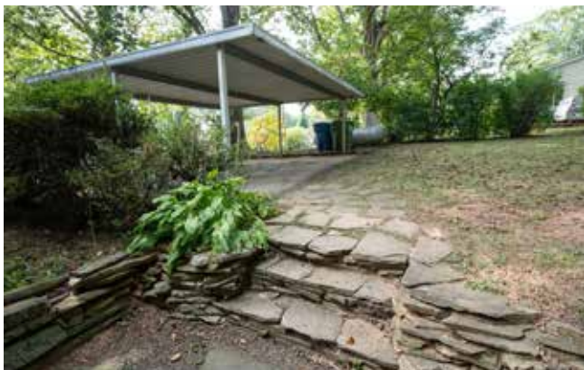
Stacked Stone Wall and Steps
