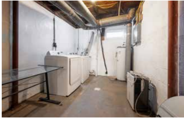
Laundry and Utility Room
