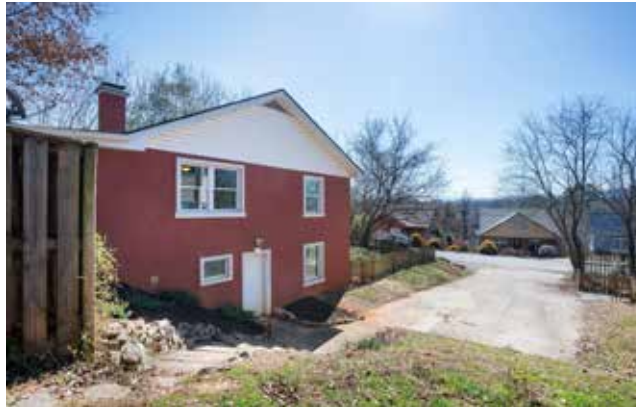
Side Entrance from Top of the Driveway
