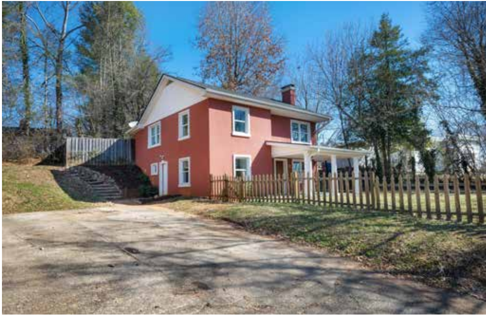
Sloped Side Yard with Stone Landscaping
