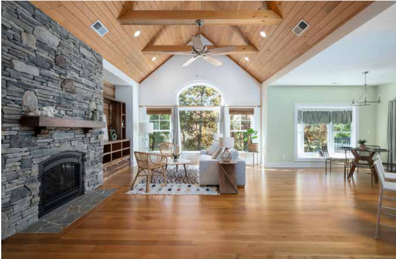
Spacious Living Room with Quarter-Sawn White Oak Floors and a Knotty Cypress Tongue-and-Groove Vaulted Ceiling
