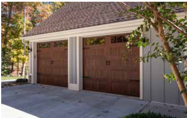
Oversized, Two-Bay Garage
