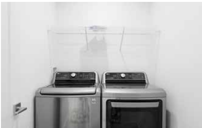
Second Laundry in Basement
