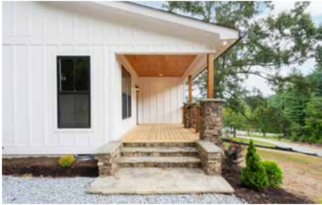
Front Entrance Featuring Real Rock® Steps
