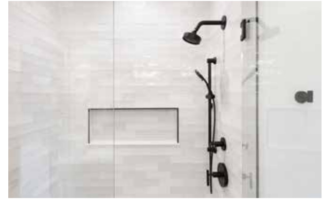
Tiled Primary Shower with Kohler® Fixture
