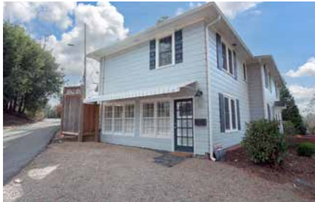
Off-Street Parking for Three
