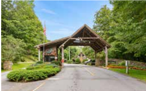
Gated Secured Entrance
