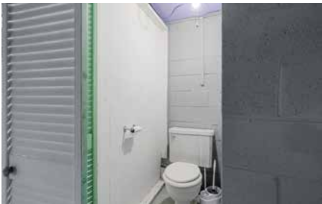
Basement Has Some Existing Plumbing
