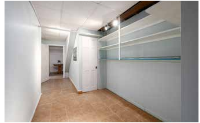
Basement Hallway off Laundry
