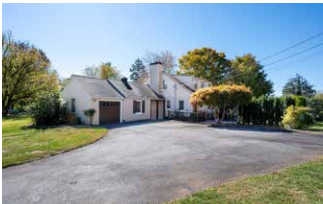
Large Driveway • One-Car Garage
