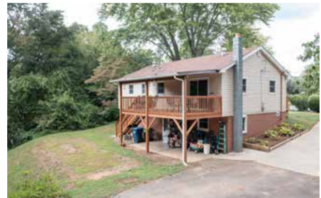
Rear View of Walk-out Basement with Covered Patio
