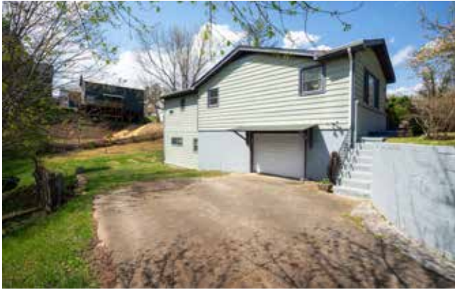
Ample Parking • Garage Access
