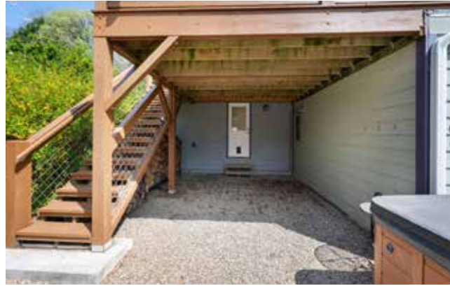
Door to Basement • Hot Tub Patio
