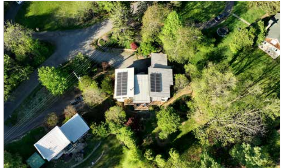
Solar Panel PV System for Low Energy Bills
