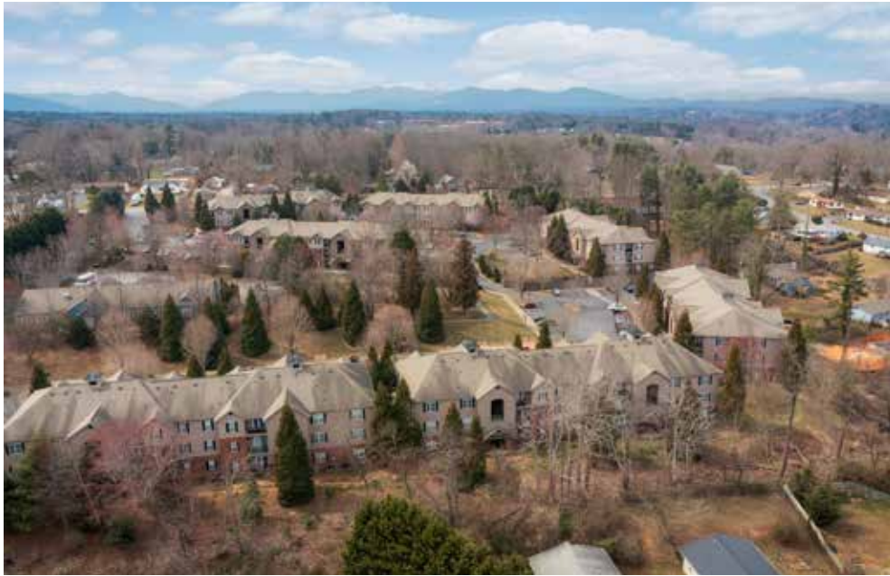
Aerial View • Long-Range Mountain Views
