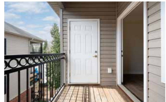
Private Balcony with Storage and Living Room Access
