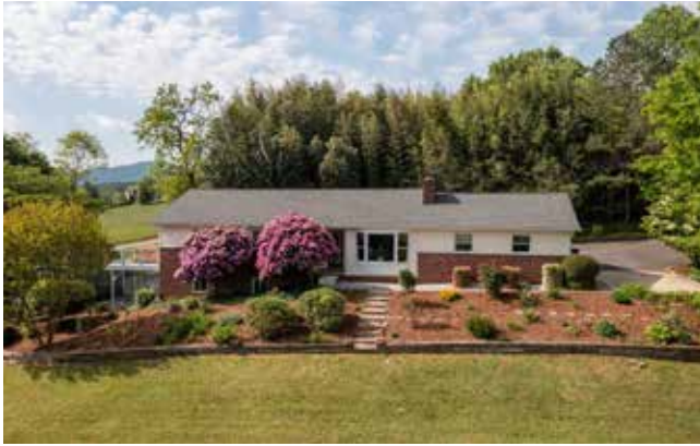
New Roof in 2020
