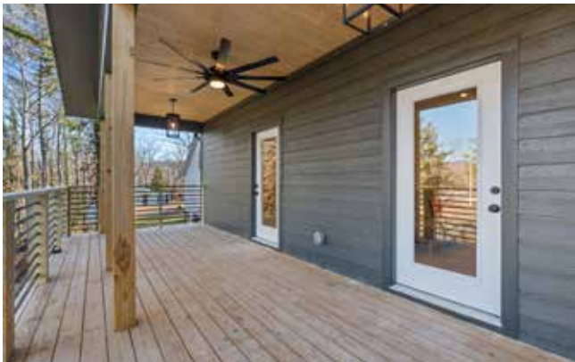
Stunning Upper-Level Balcony ...
