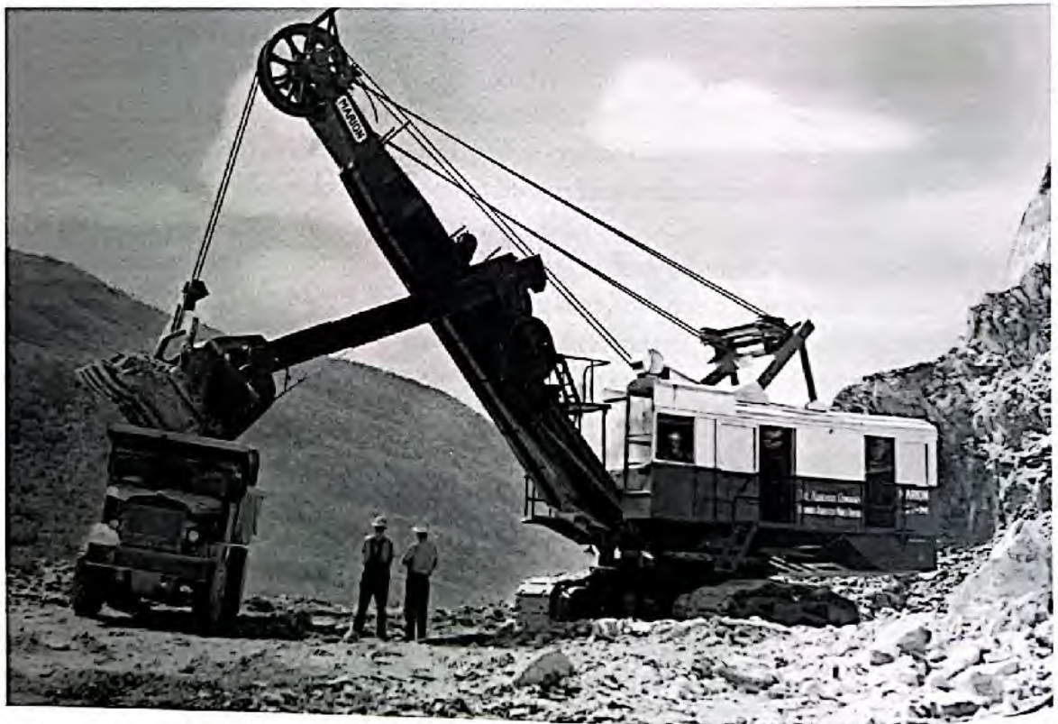
The large Marion shovel could move 50 tons of material at once.
