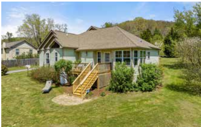
New, Rebuilt Exterior Stairs
