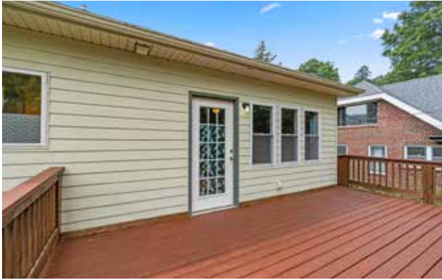
Low-Maintenance Siding on Addition
