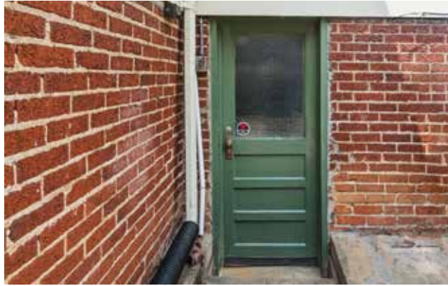
Access to Basement from Driveway
