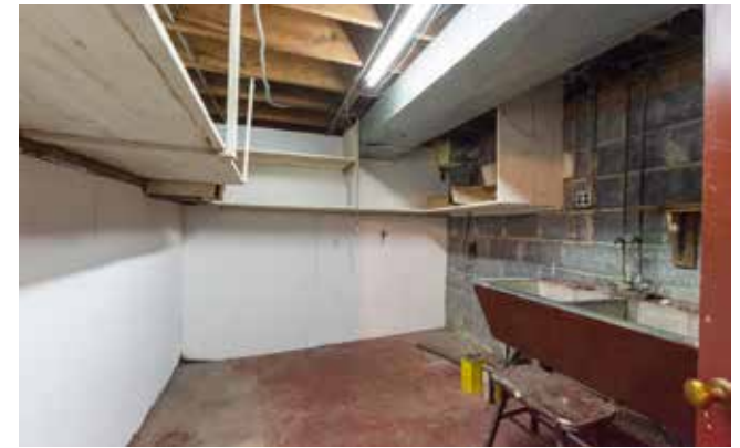
Laundry Room with Large Utility Sink
