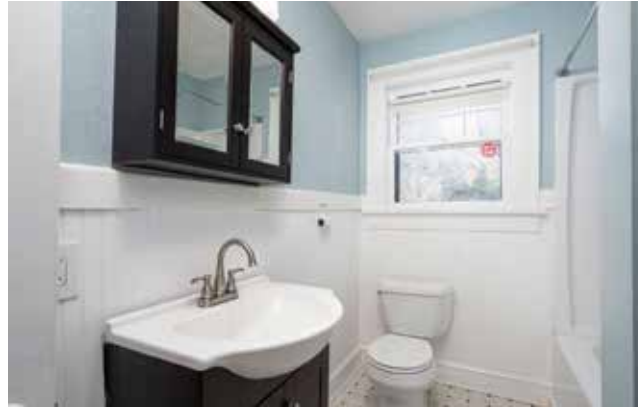
Bathroom with Newer Vanity and Protective Wainscoting
