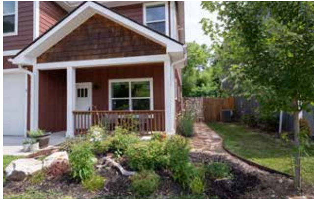
Hardieboard Siding and Cedar Shake Shingles
