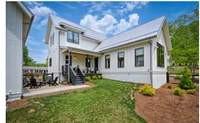
Metal Roof, Board-and-Batten Siding
