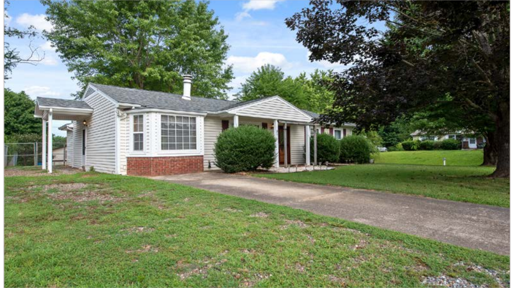
Separate Entrance to Converted Garage
