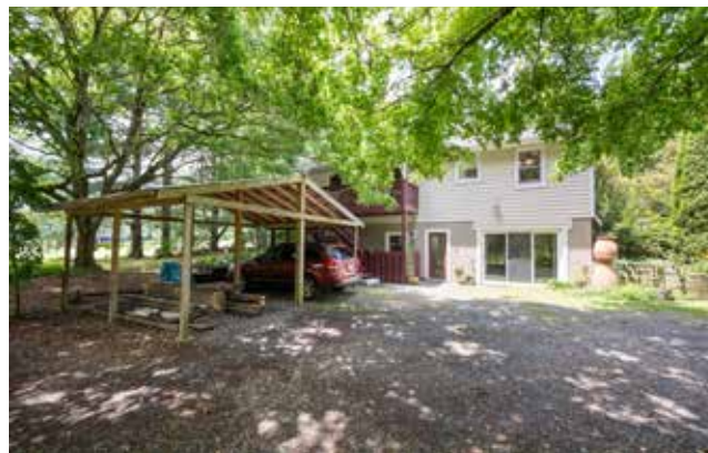
Covered Carport with Metal Roof
