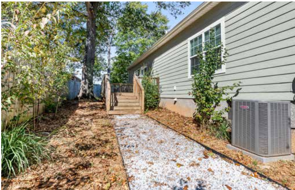
Back Deck and Walkway
