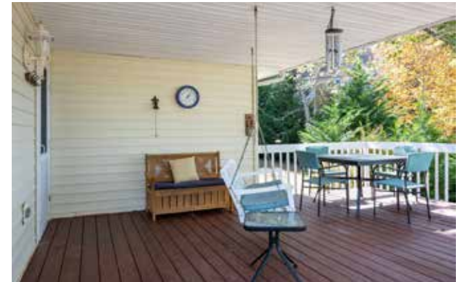
Partially Covered Deck
