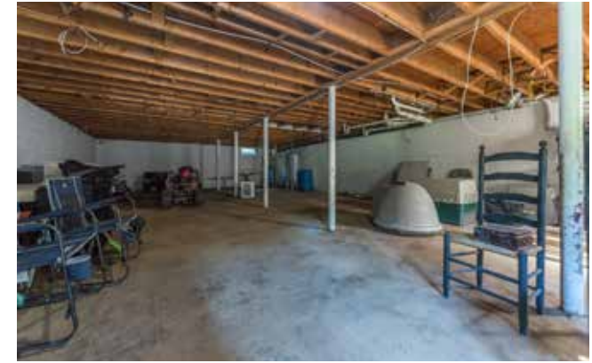
Large Unfinished Basement
