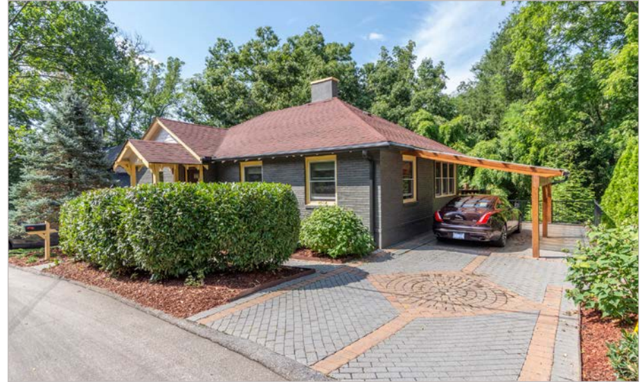
One-Car Carport and Paved Driveways
