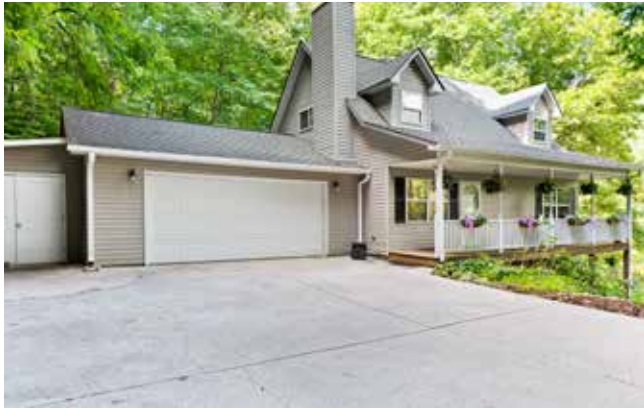
Attached, Two-Car Garage
