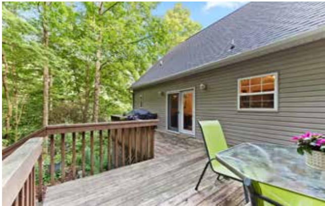
Deck Is Accessed via the Kitchen ...
